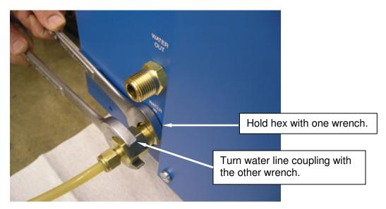
Figure 11 Connect and Remove the Water Lines
